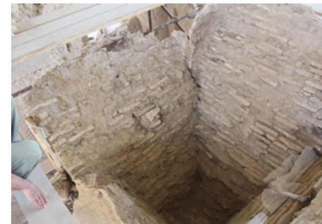
88. View of the technique by which the intersection among different arcades is solved.
