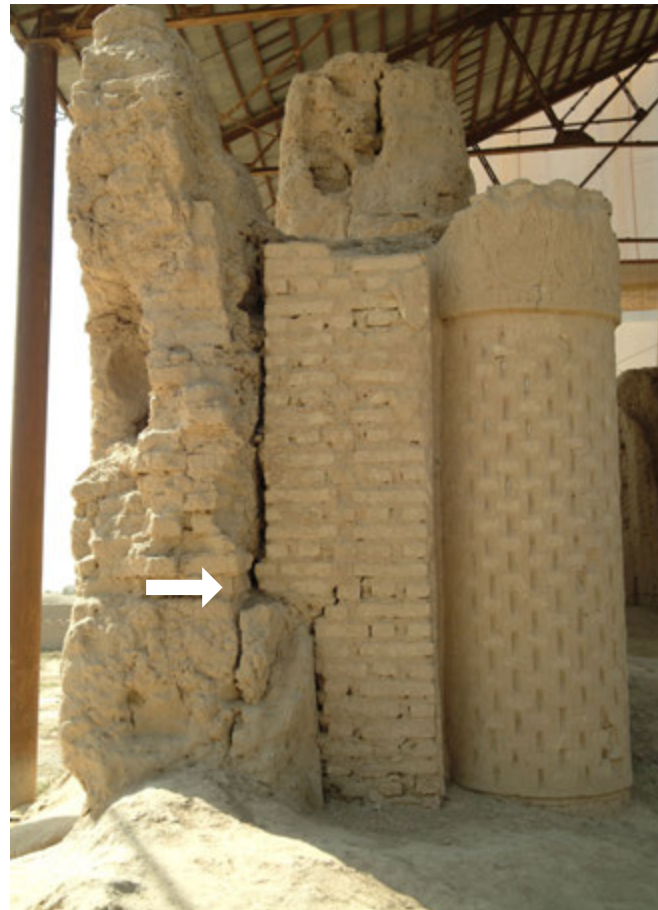
2. Section of the south wall. The arrow shows the pakhsah structure relating to the first mosque.
