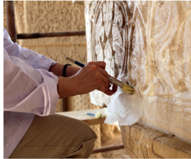
27. Applying hemp paper for facing.
