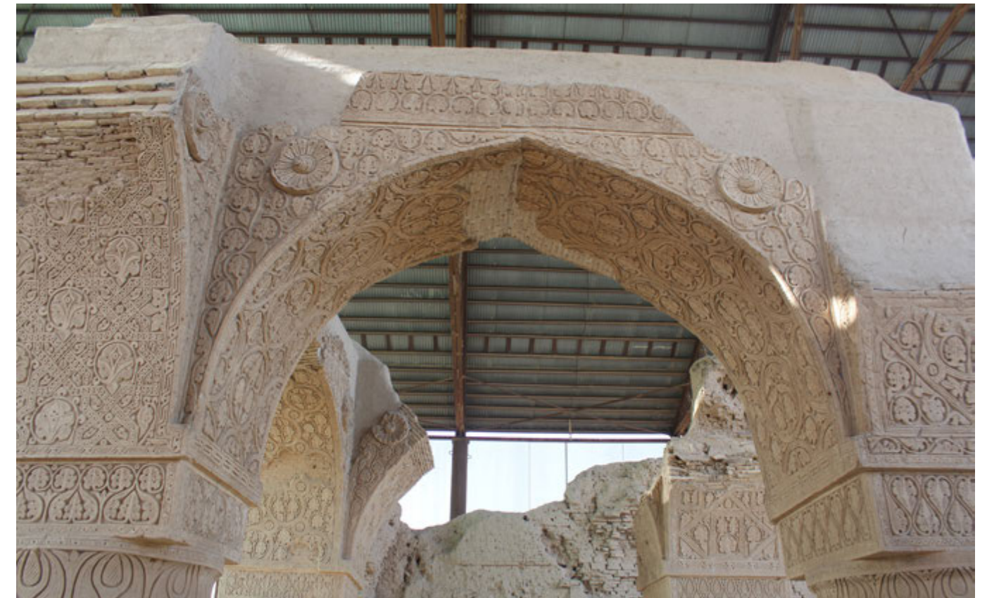
105. View of the arch 6–10, seen from south, after consolidation.
