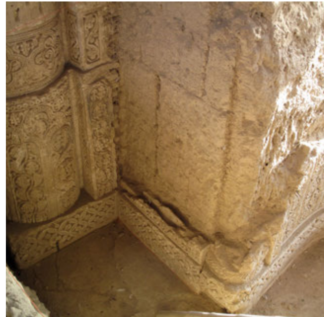
76. West wall, mihrab .
