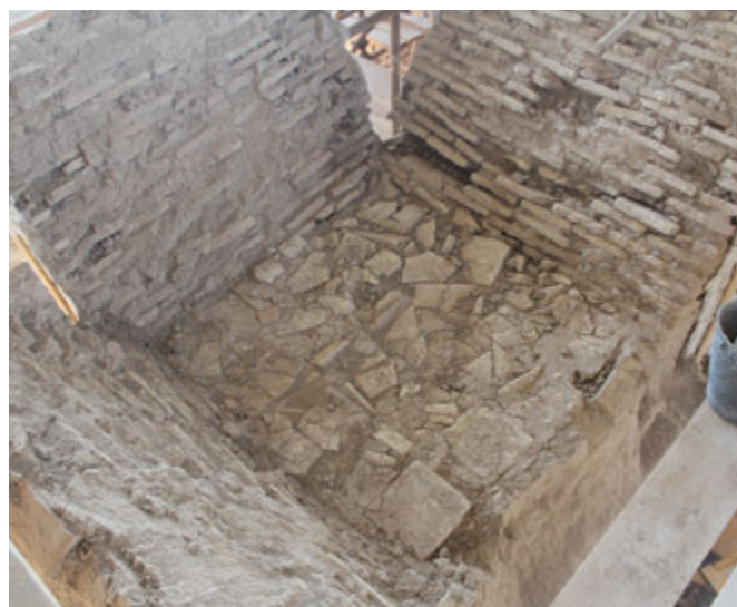
89. The rough filling material.
