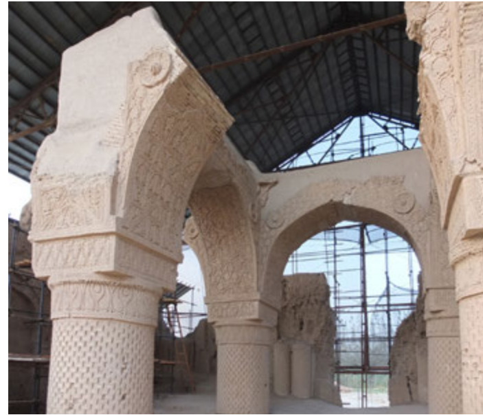
107. The arch system (6-10 and 10-11) looking from east, after consolidation.
