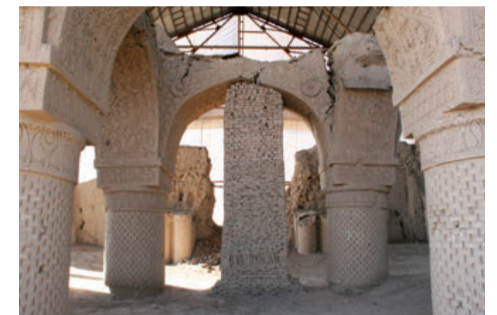
1. General view of the two standing arches (2007).
