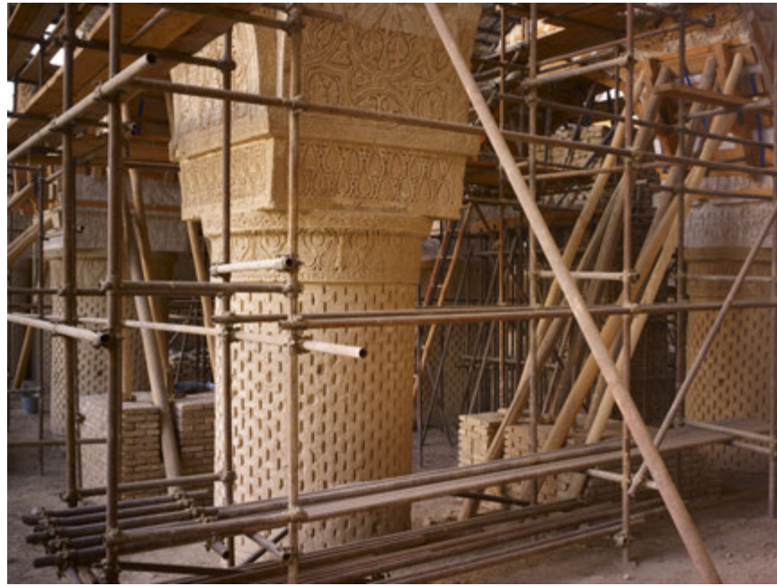
1. View (during conservation) of springing of arches between columns 7 (foreground) and 11 (direction west), showing multiple designs of decorated stucco relief at column head and arch soffit.
