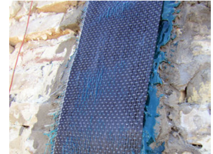
23. Applying carbon fibre strips on top of epoxy resin.
