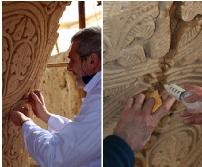
26. Cleaning and consolidation of the plaster decoration.
