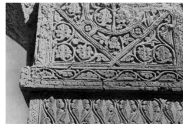
18. Soffit and impost block of soffit 5-6, pillar No. 6.
