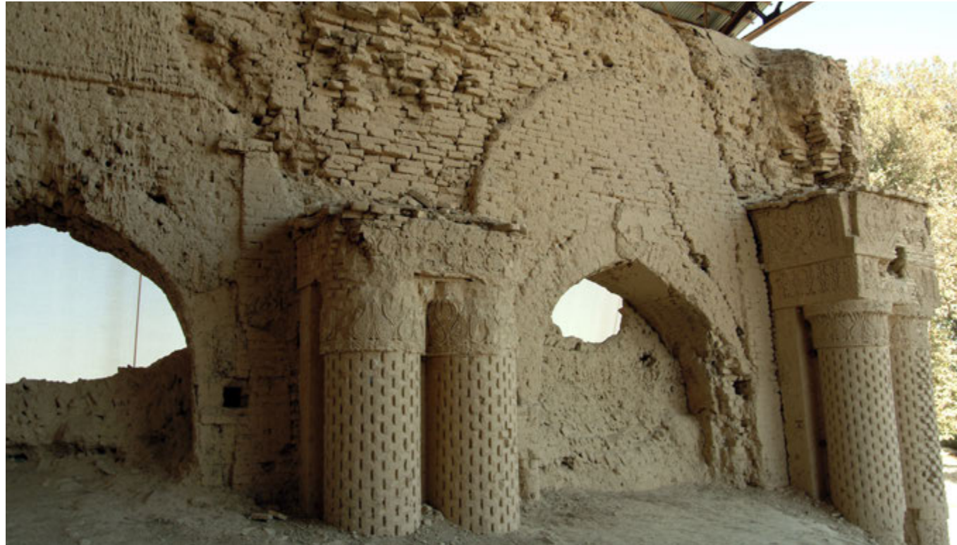
86. Internal view of north wall.
