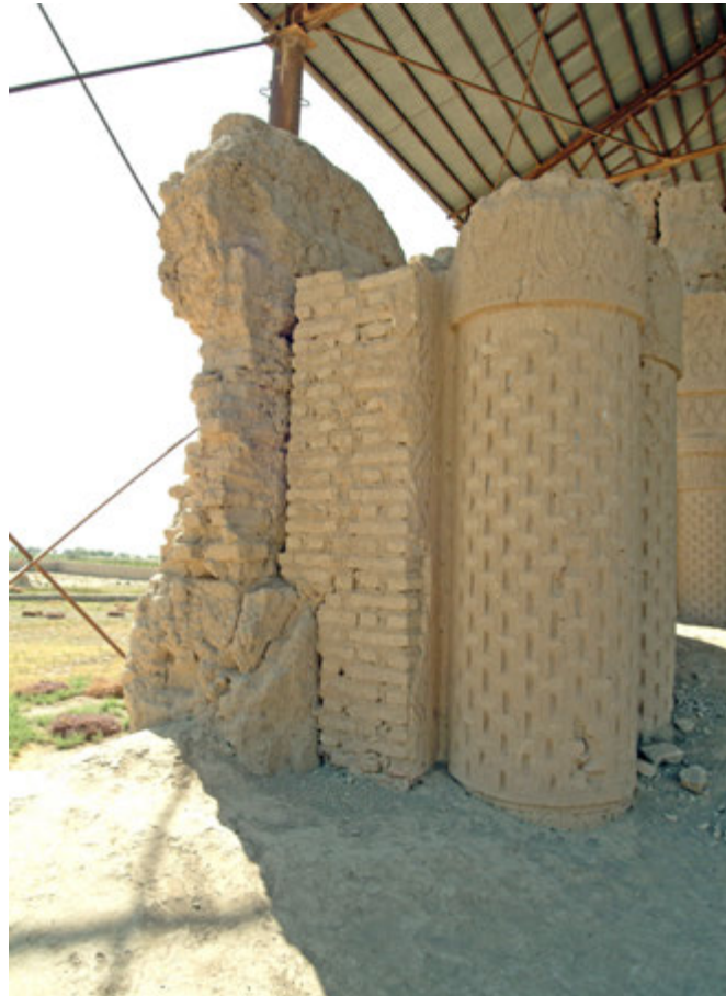
75. South wall, looking from the east.
