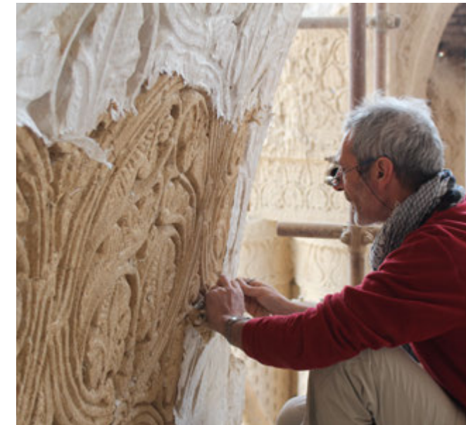
69. Removing the facing.
