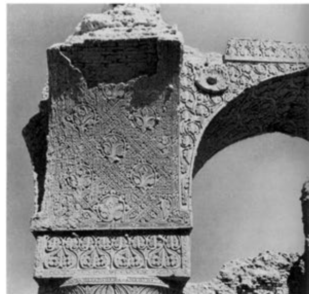
13. Soffit 9-10, pillar No. 10.
