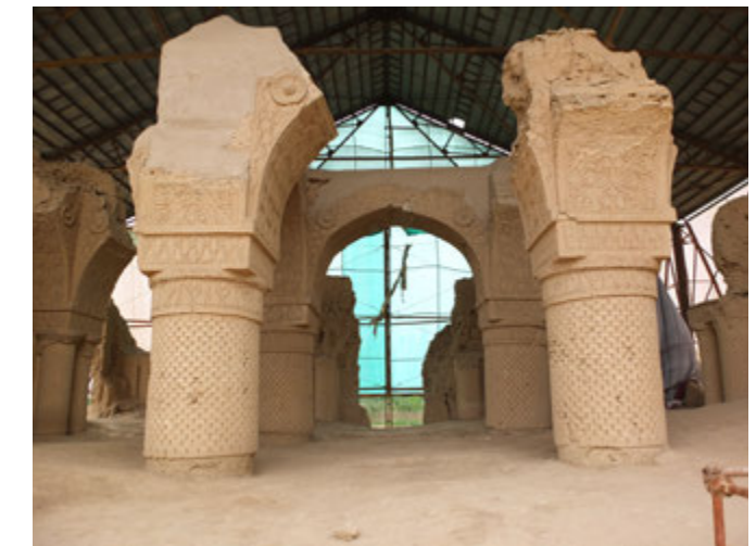
71. General view of the arches after consolidation.
