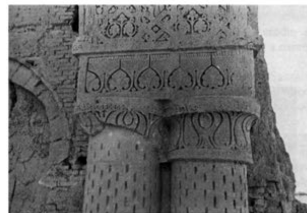
15. Columns, capitals, and impost block of No. 9.
