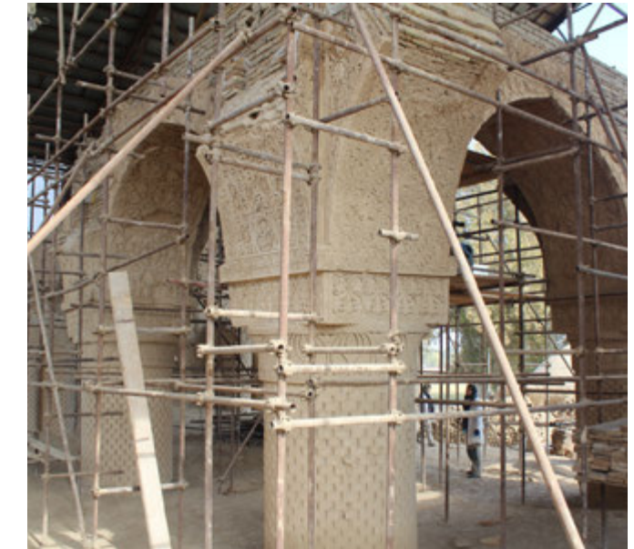
70. General view of the consolidated arches before mud plaster application.
