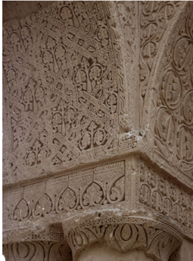
4. The distinctive characteristic of the carved stucco ornament is the association of compartments designed as geometrical figures, defined by thin framing bands, with stylised vine leaves.
