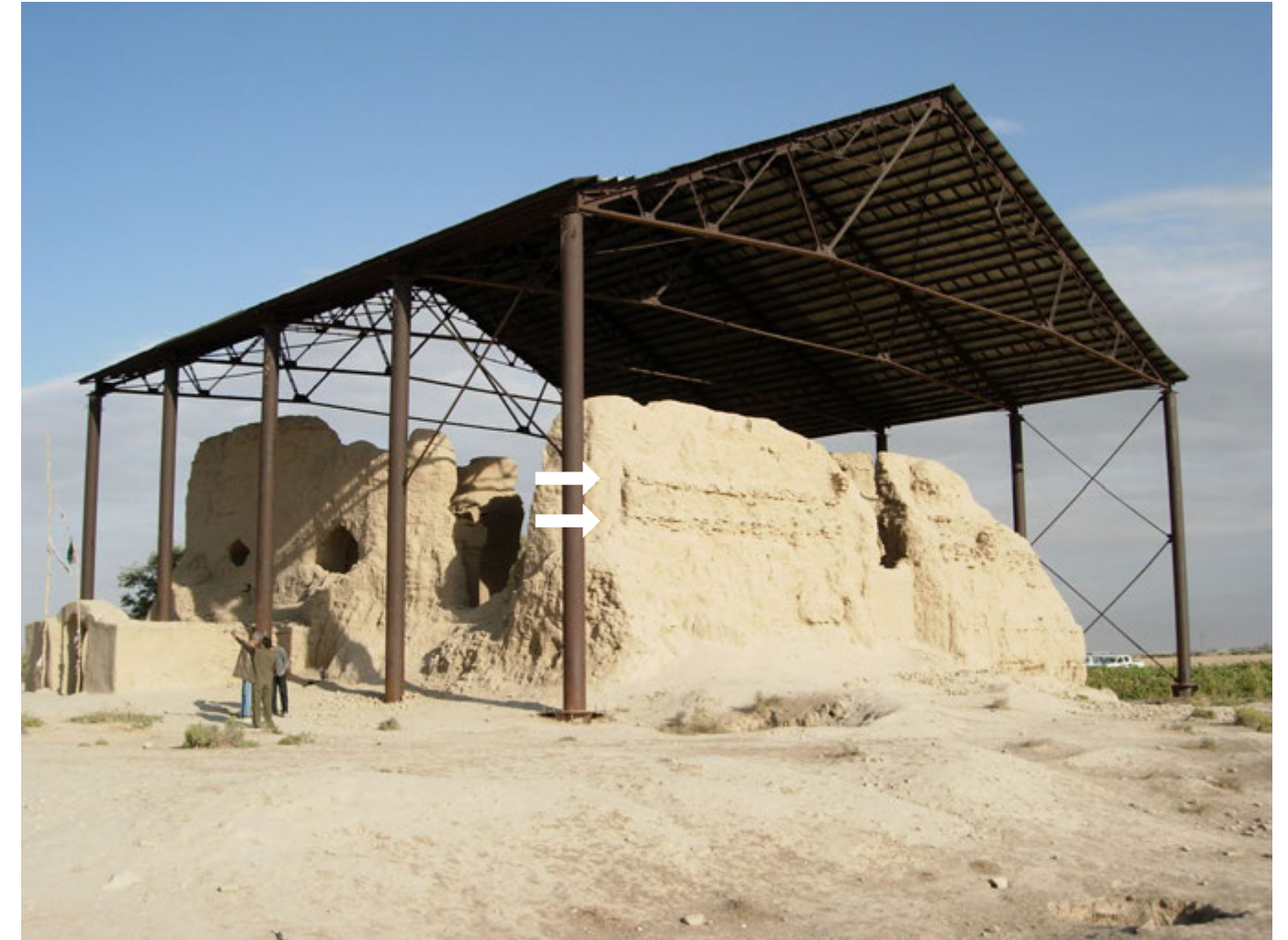
5. View of the qibla wall with (arrows) the courses of baked bricks.
