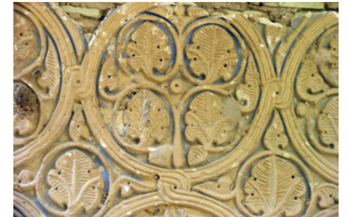
10. The effect of lapis lazuli blue at the base of the decoration.
